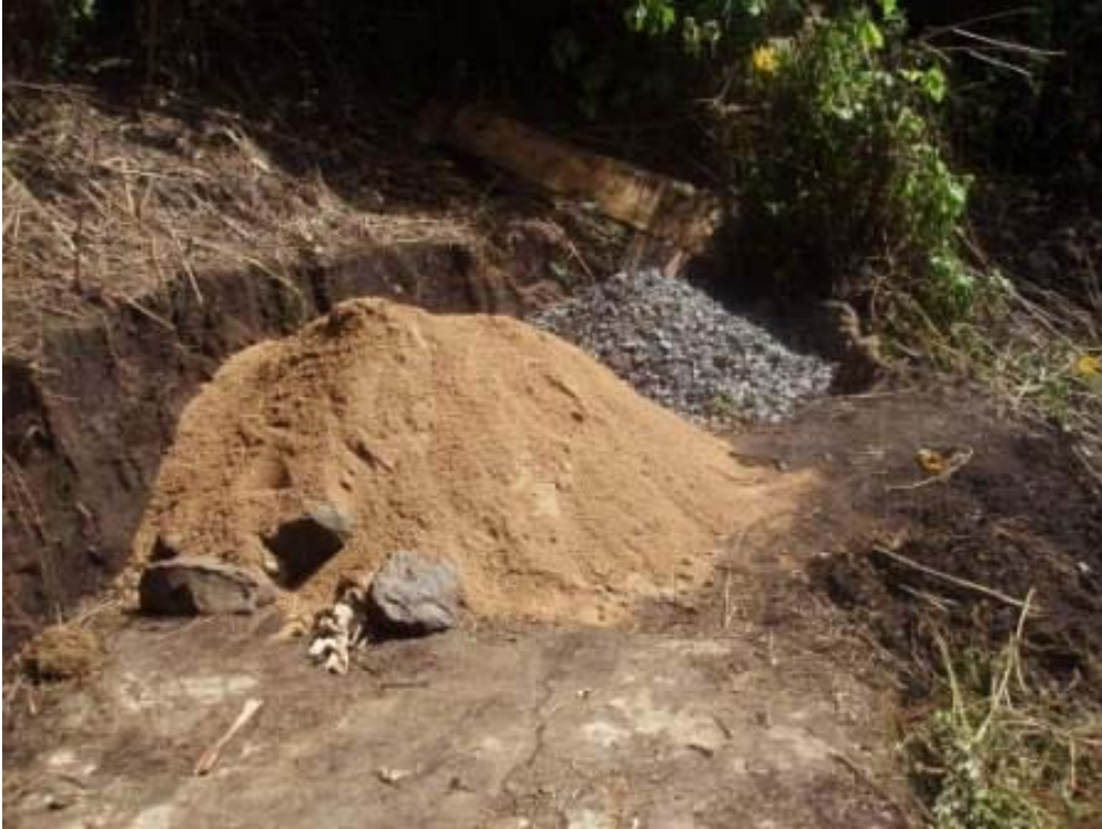
Sand and stones left to continue the water distribution system
