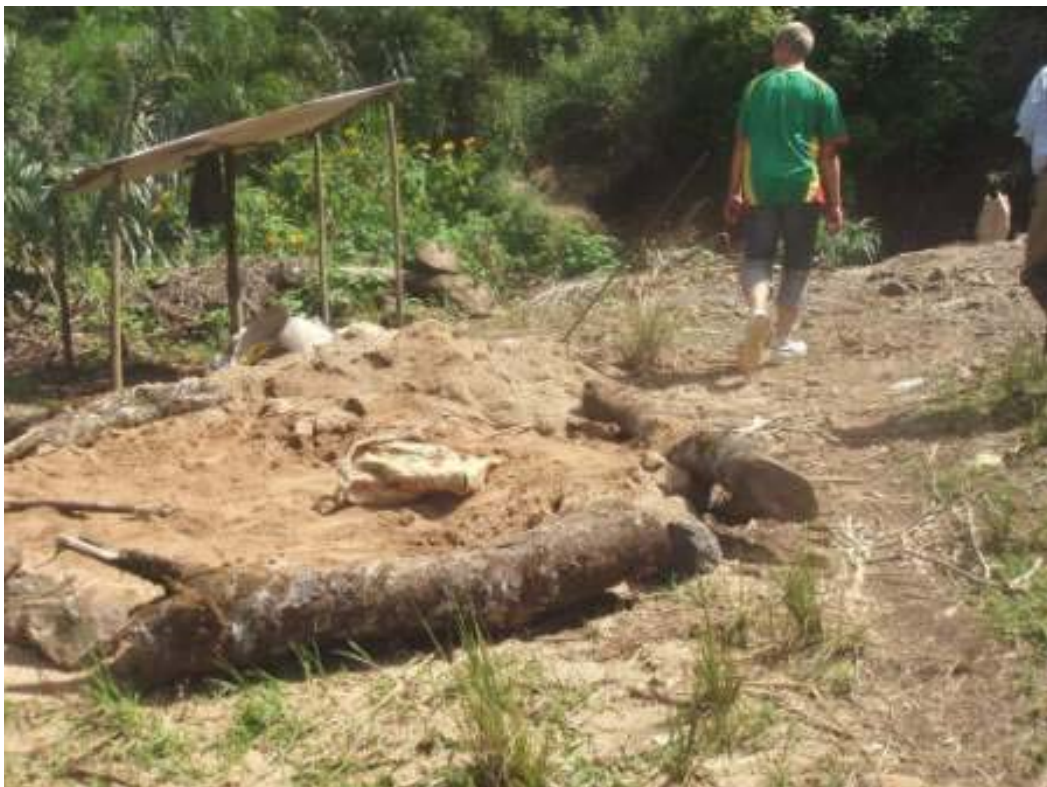
Newly built spring catchment site
