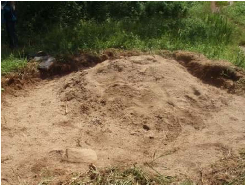
SAND USED FOR WORK at project site
