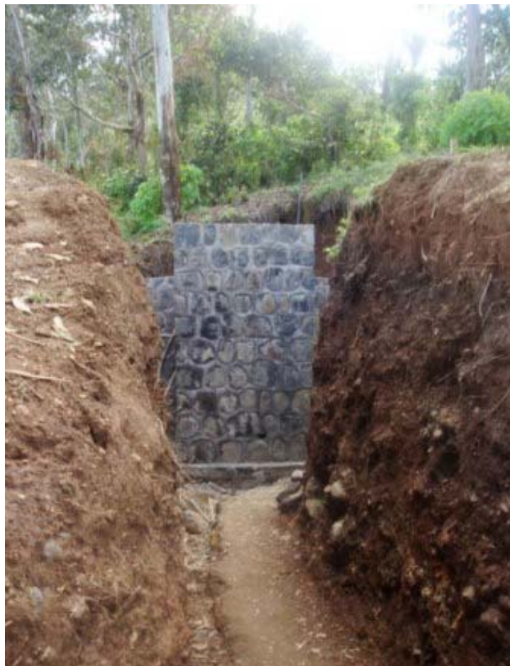
Entrance to the 10,000 cubic meters water tank
