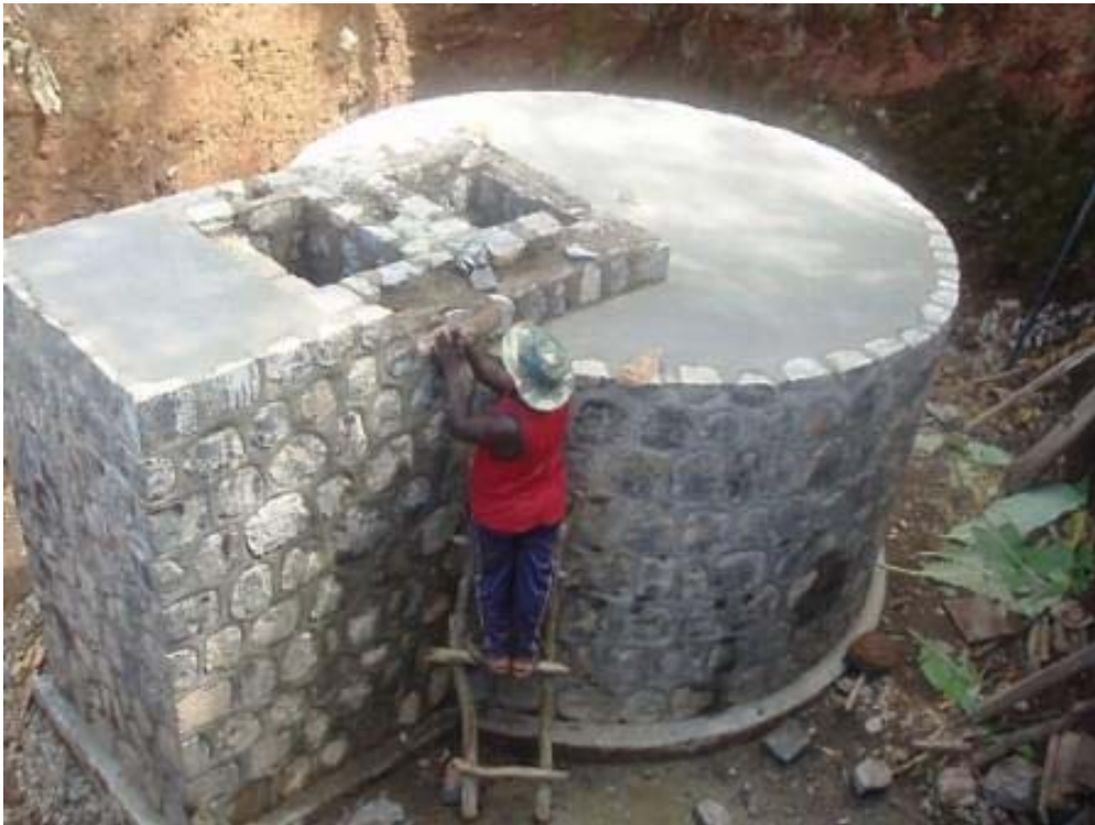
Upper view of the tank
